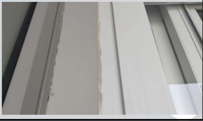
Sliding door frame and switch board packing and cleaning the border area to get proper finishing .
