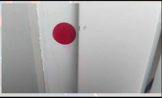
Major scratch marks found on the left side sliding door frame .
