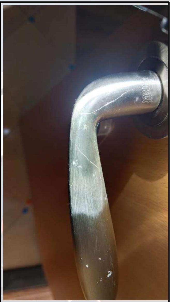
Scratch marks found on the door handle .
