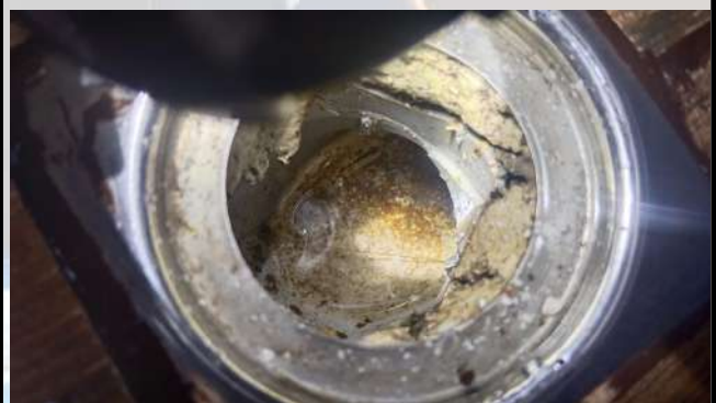
Drainage pipe inside proper packing finishing required as well as cleaning .
