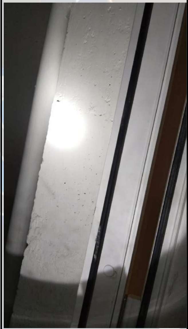
Window external side plaster finishing not proper and cleaning required
