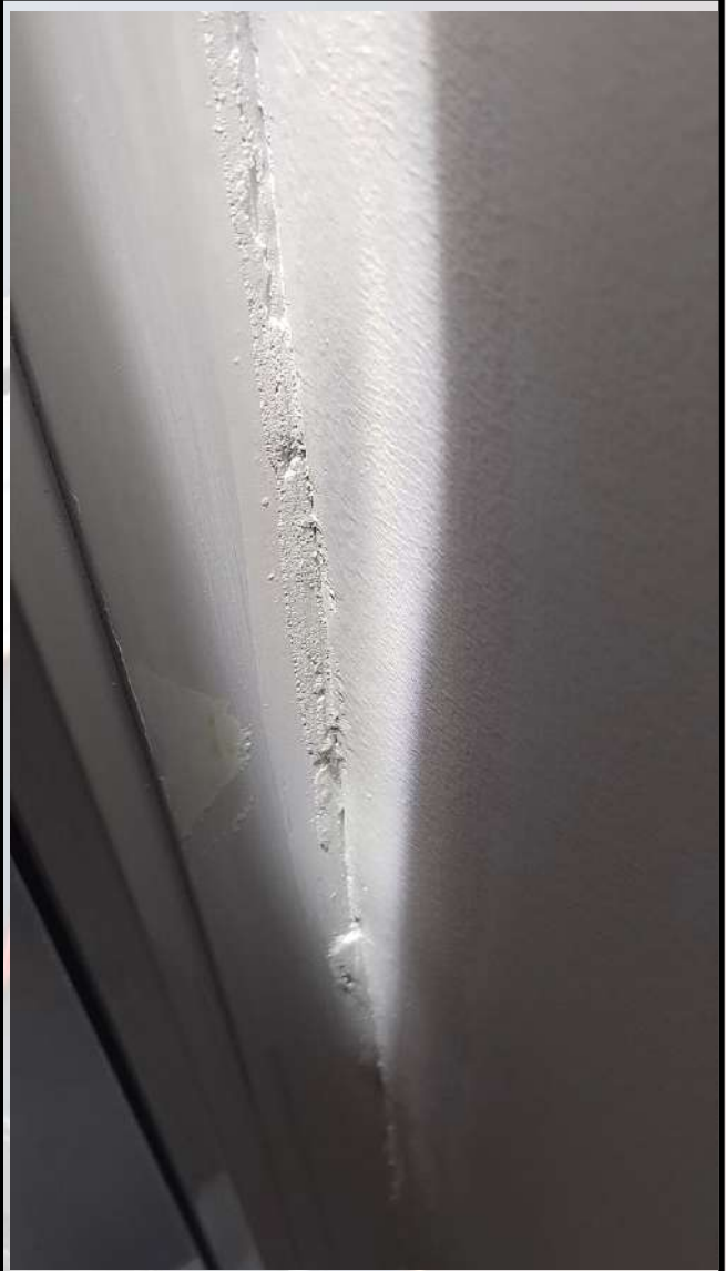
Window frame packing finishing not proper ,proper finishing required .
